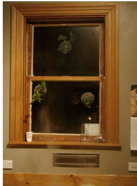
Pod linings installed on kitchen window
