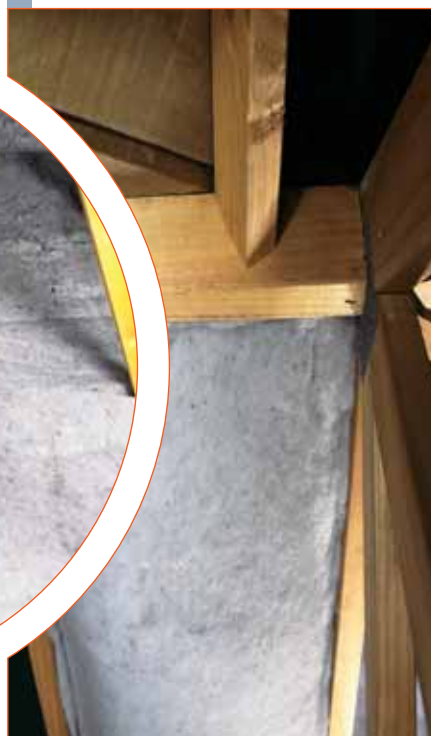
6 Completed exposed rafter job
