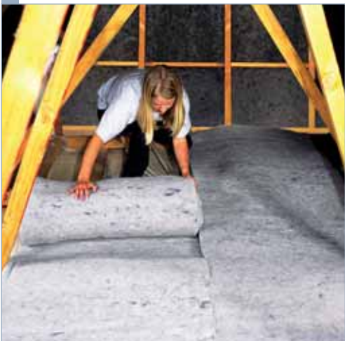
2 Rolling out over framing
