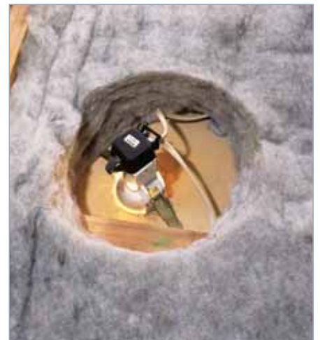
4 Clearances around down-lights
