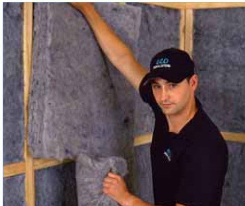
1 Fitting to wall cavity
