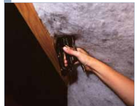
7 Additional support to rafter installation
