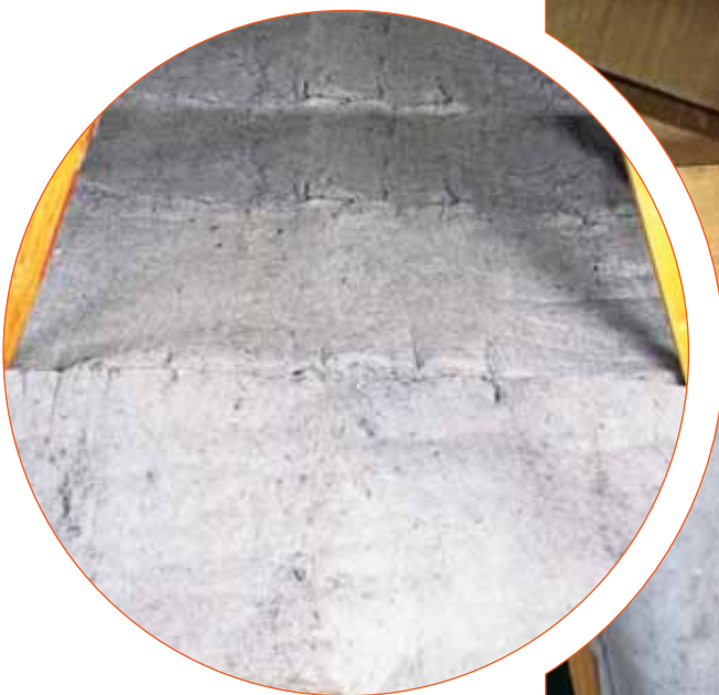
5 Completed attic ceiling
