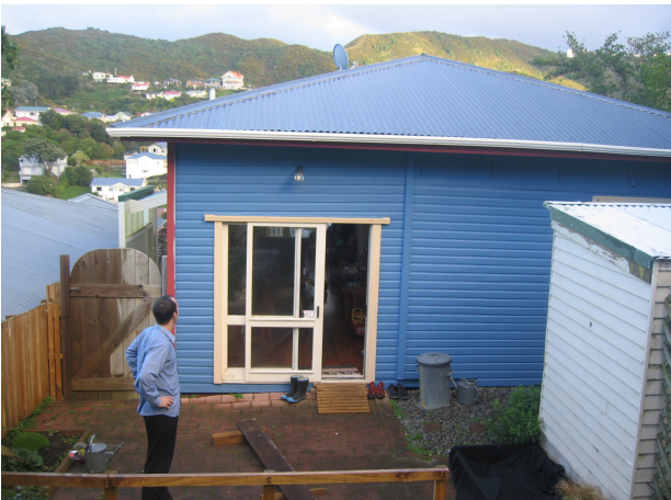
Rear of Existing House
